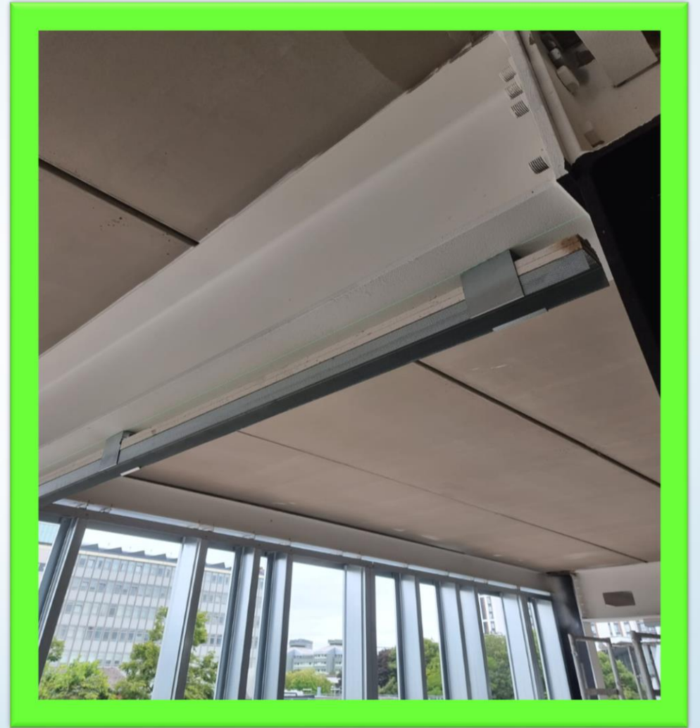
Installation with HTC
